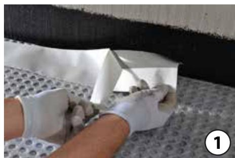
2. Lay **PROBAND BU** on the bituminous covering, PVC, wooden, polycarbonate, glass, plastic or metal.
