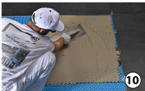
11) Apply the same adhesive, onto the wet one, using a notched trowel according to the tile size.
