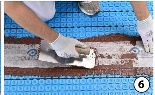
**Warning:** PRODESO HEAT GRIP 5 is not a waterproofing membrane; to get a proper waterproofing for indoor environments, after installation of the heating cable, you have to do the following:
