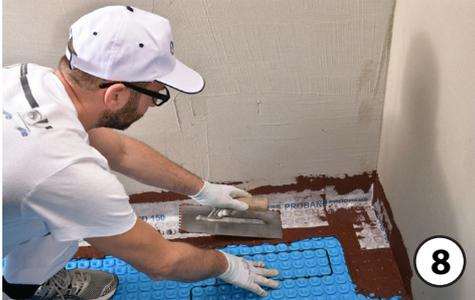
11. Apply adhesive on the back of the tiles using a 3 x 3 mm notched trowel to guarantee the full coverage and a thickness above the heating cable of at least 5 mm.
